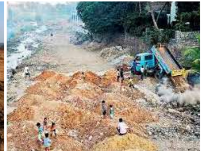
Construction Work On /Around Pond
