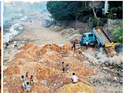
Construction Work On /Around Pond
