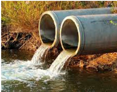
Discharge of Sewage
